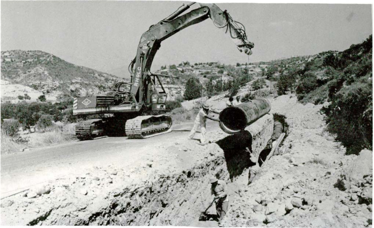
Kalavassos-Khirokitia Pipeline. Installation of 900 mm dia pipeline. WDD Photo E57-9 (5.9.84).
