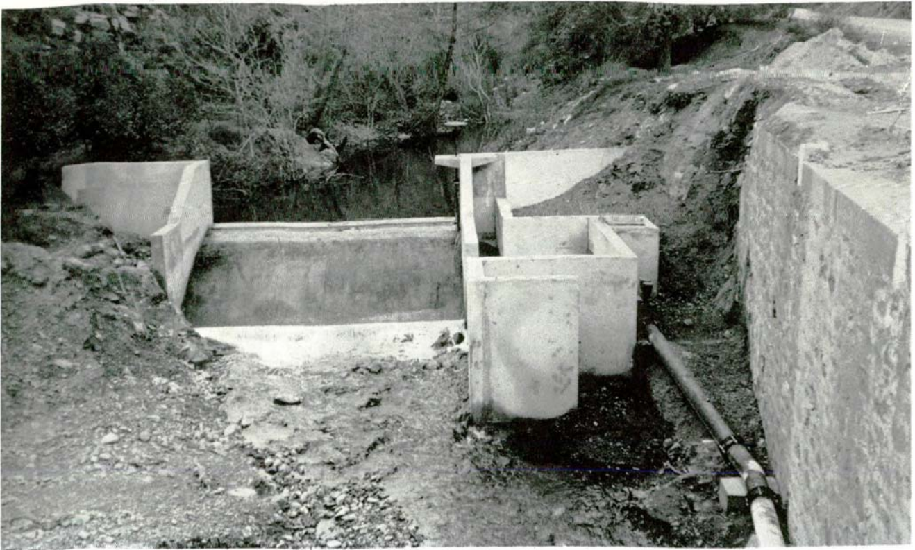
Pitsilia Integrated Rural Development Project. Diversion weir serving Dhierona and Arakapas No. 2 Ponds. WDD Photo E15-8 (20.2.84).
