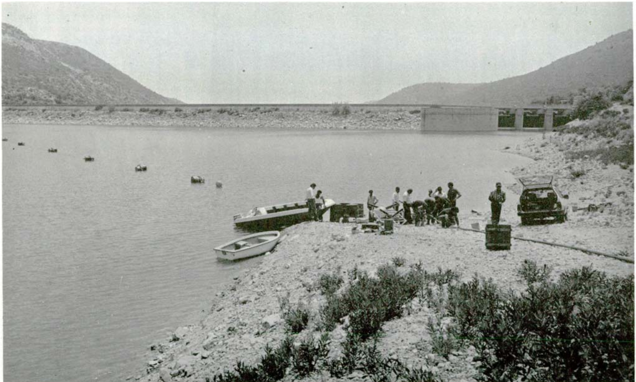
Yermasoyia dam. Reservoir aeration. WDD Photo D58-3, 24.5.83.
