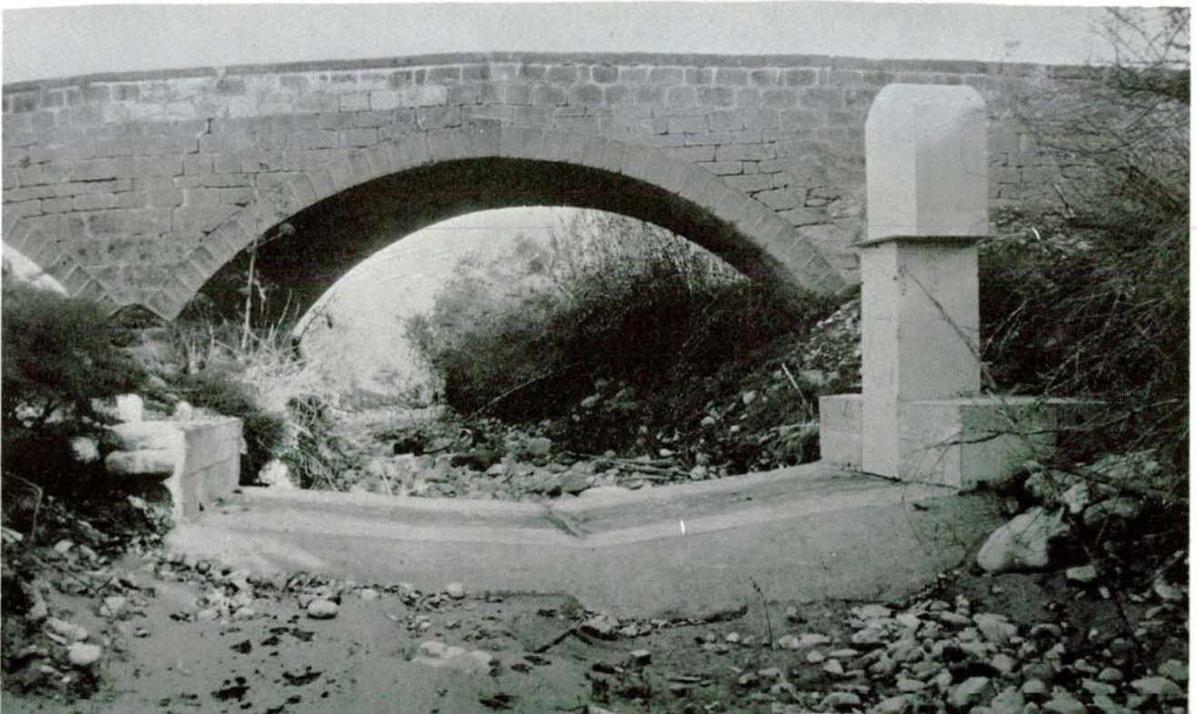
A weir established upstream the sinkhole area near Maroni village to record the inflow into the aquifer through the sinkholes. WDD Photo E4-9, 4.1.84.
