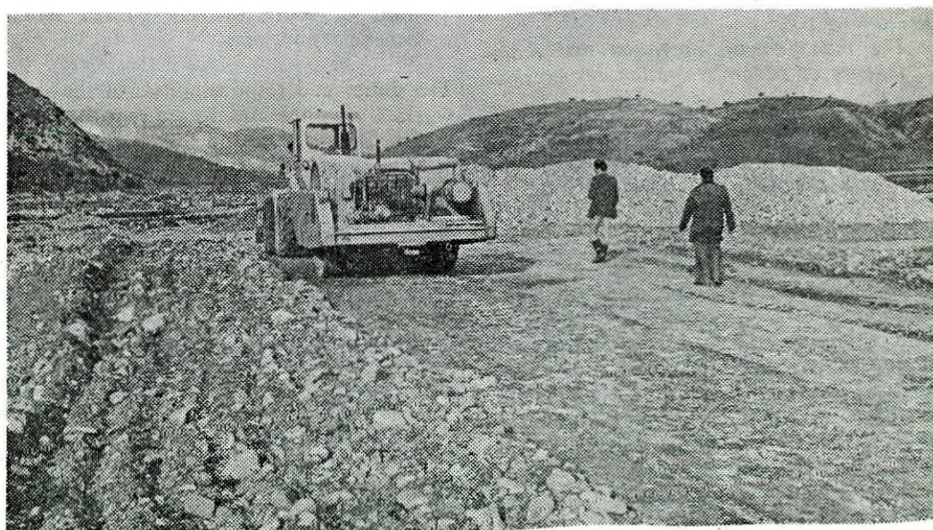
Compaction Tests Carried out at Asprokremmos Damsite
