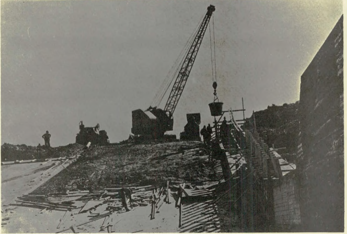
Spillway construction at Massari dam
