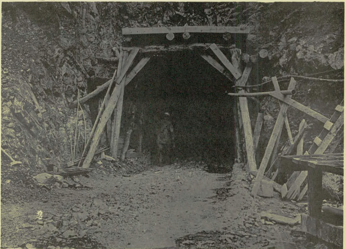
Diversion tunnel at Lefkara dam
