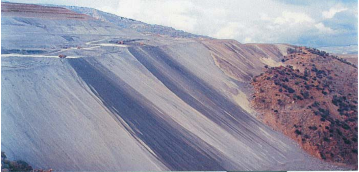
FIGURE 6. Stabilization of the Loumata valley tips.
