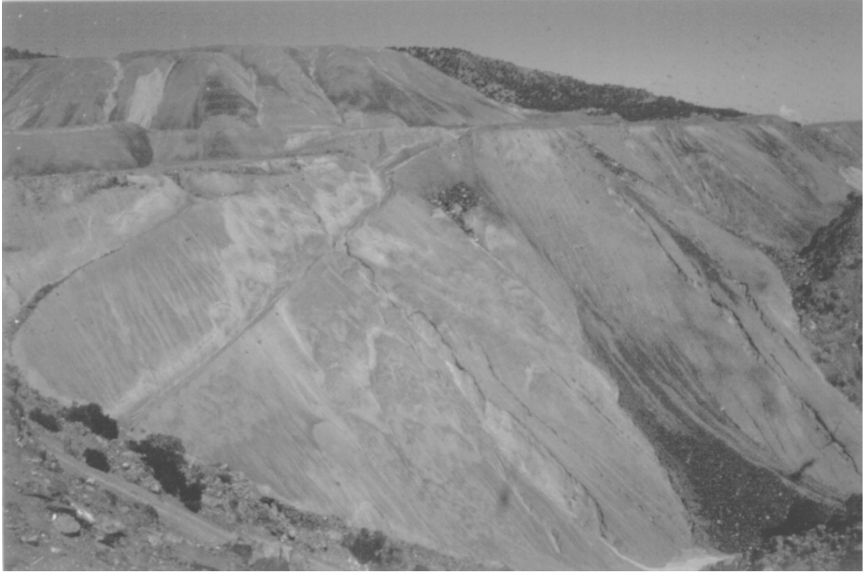
FIGURE 2. Waste tips dumped on steep slopes and side valleys.
