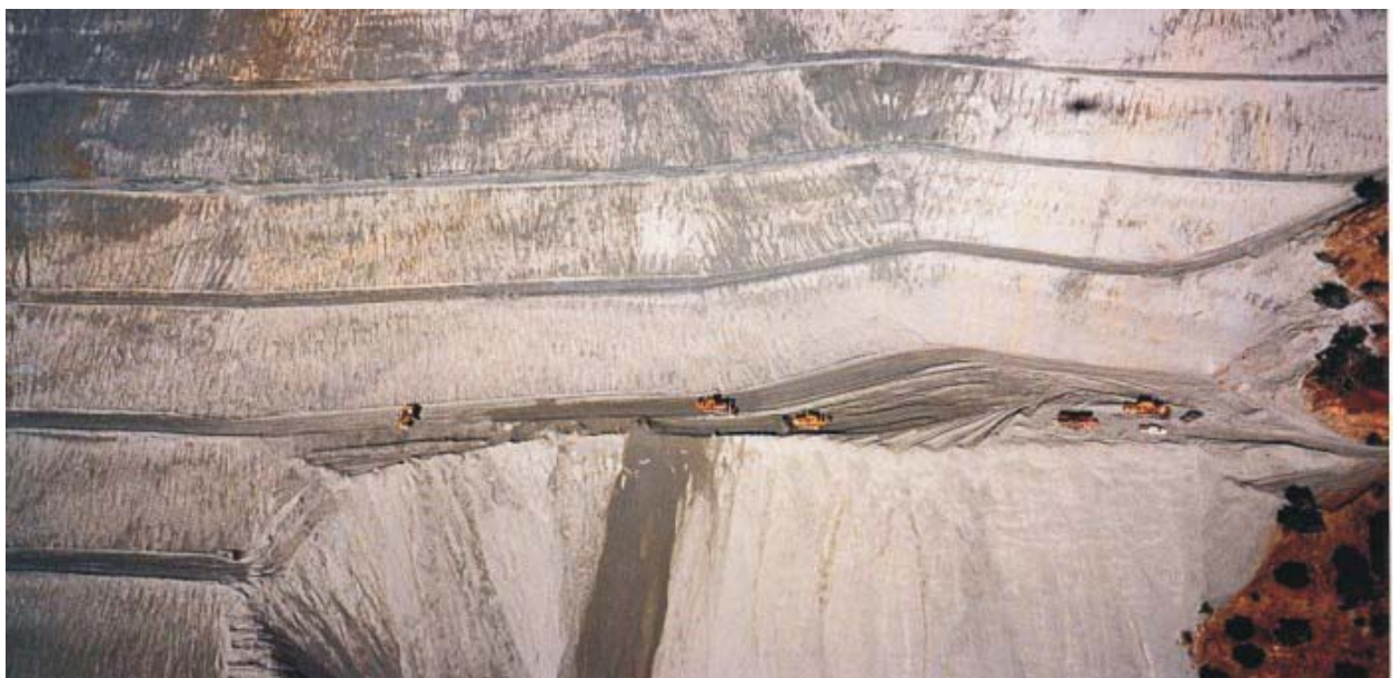
FIGURE 5. Stabilization of the Loumata valley tips.
