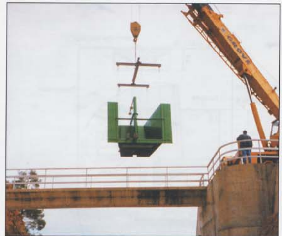
A fusegate being lowered into place.
