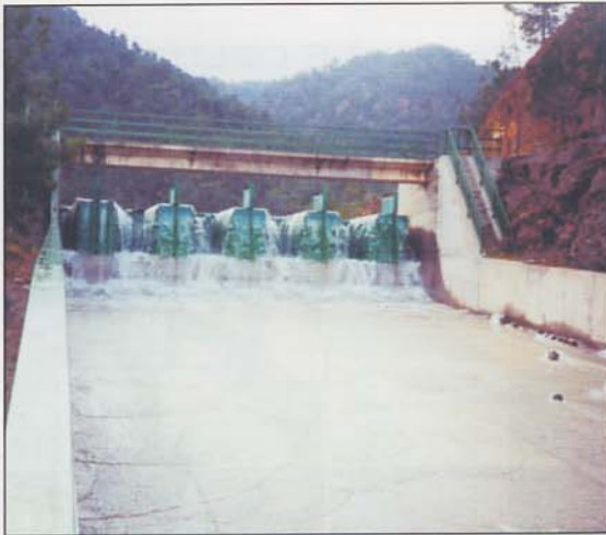
The fusegates overspilling.
