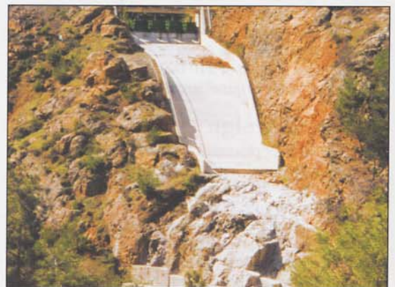
General view of the Xyliatos spillway.
