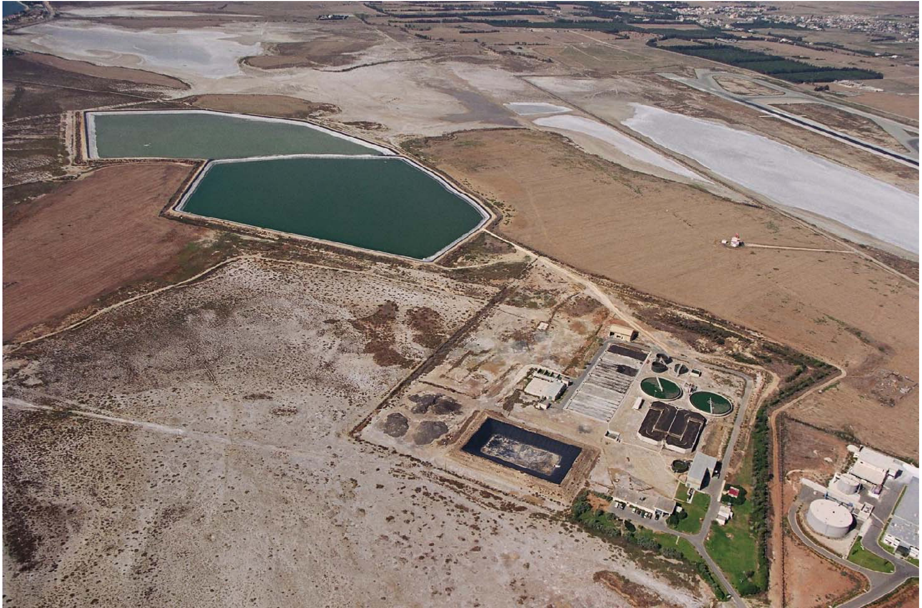
SDBL LARNACA PLANT (AIRPORT)
