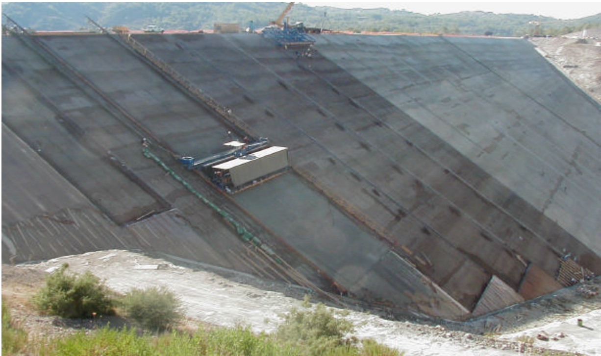
Photo.1 Upstream Face Slab Concreting
