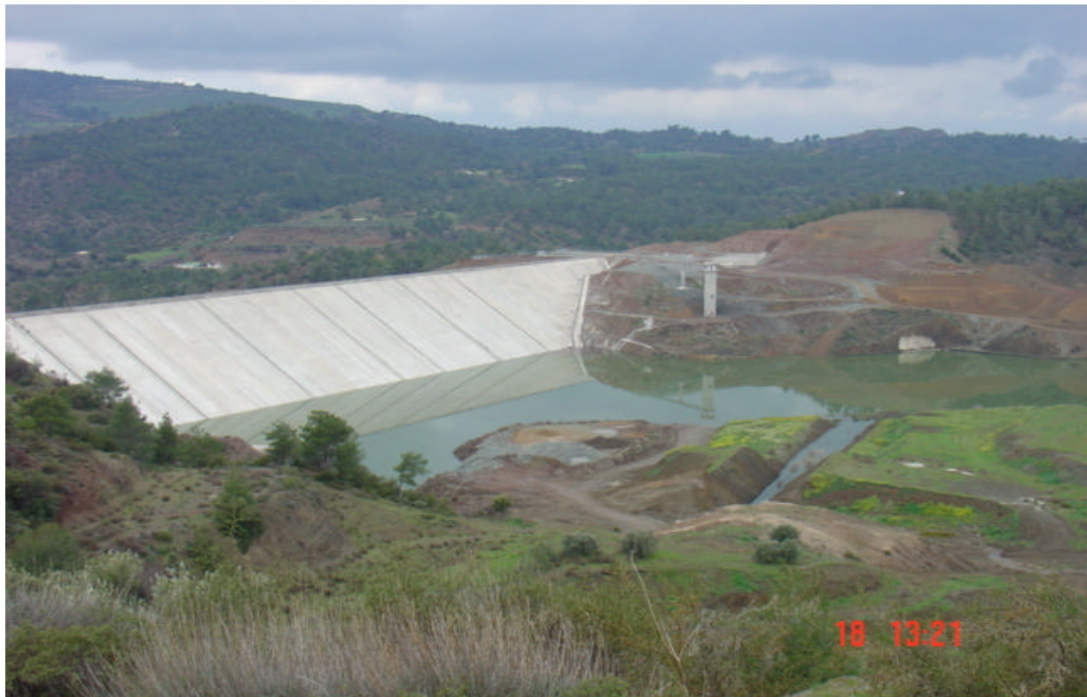
Photo 2. General view of the completed Dam
