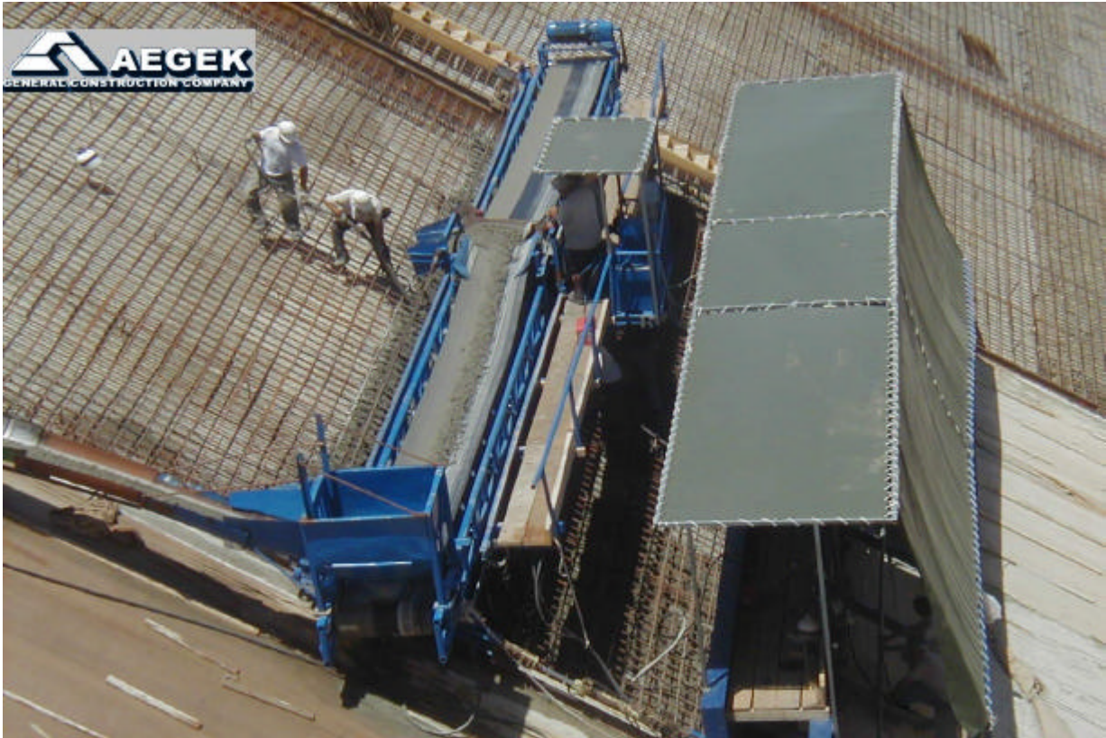
Photo 2. Self climbing slip form with side discharger
