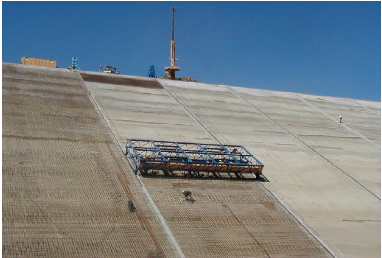
Photo 3. Reinforcement placing trolley
