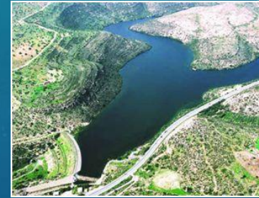
Polemidia Dam Capacity: 3.4 MCM Year: 1965
