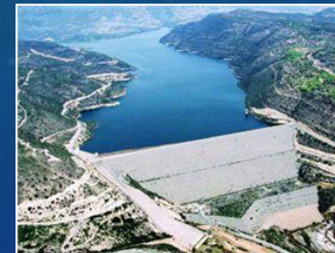
Kouris Dam Capacity: 115.0 MCM Year: 1988
