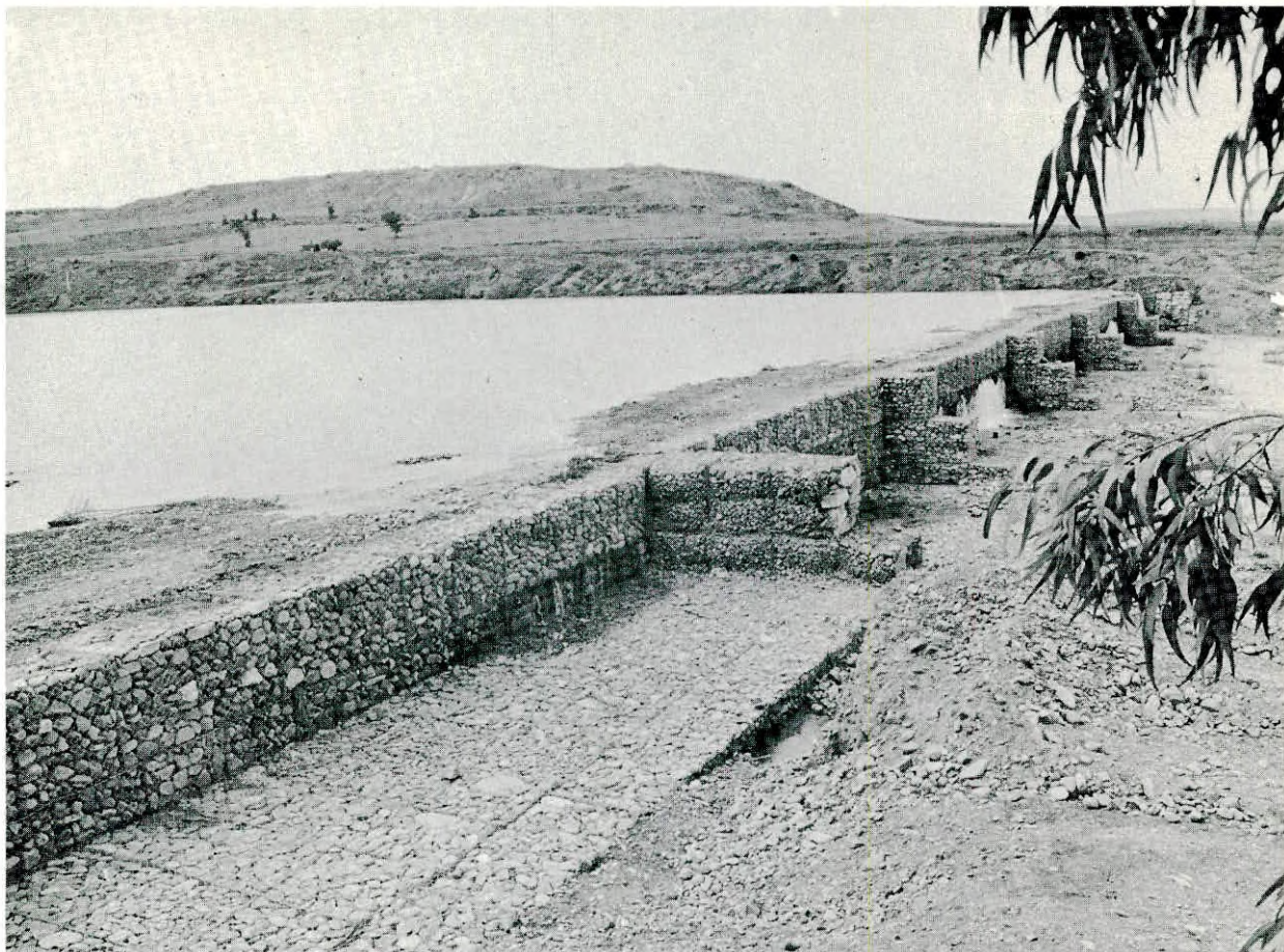
Gabion Weir for recharge purpose on Yialias river at Potamia village
