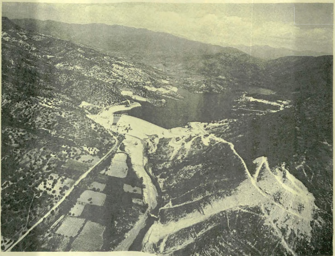
GENERAL VIEW OF YERMASOYIA DAM
