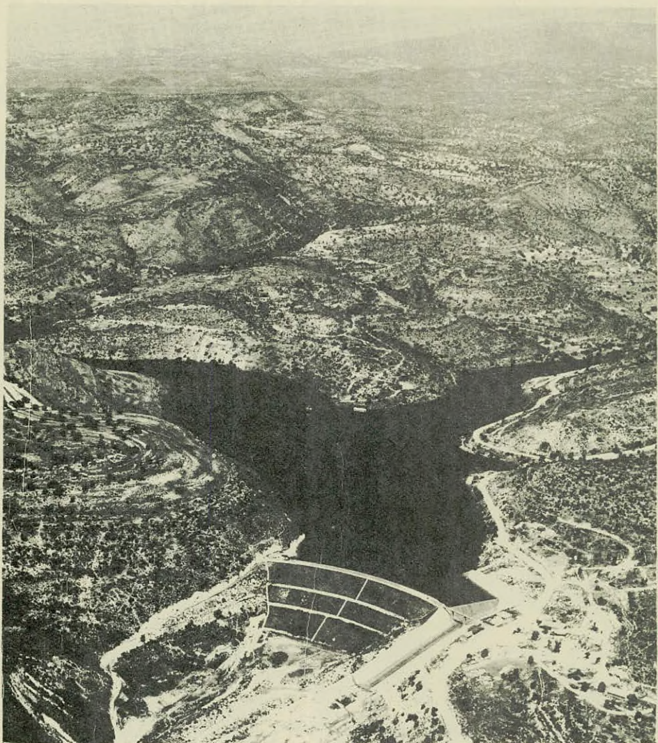
GENERAL VIEW OF POLEMIDHIA DAM
