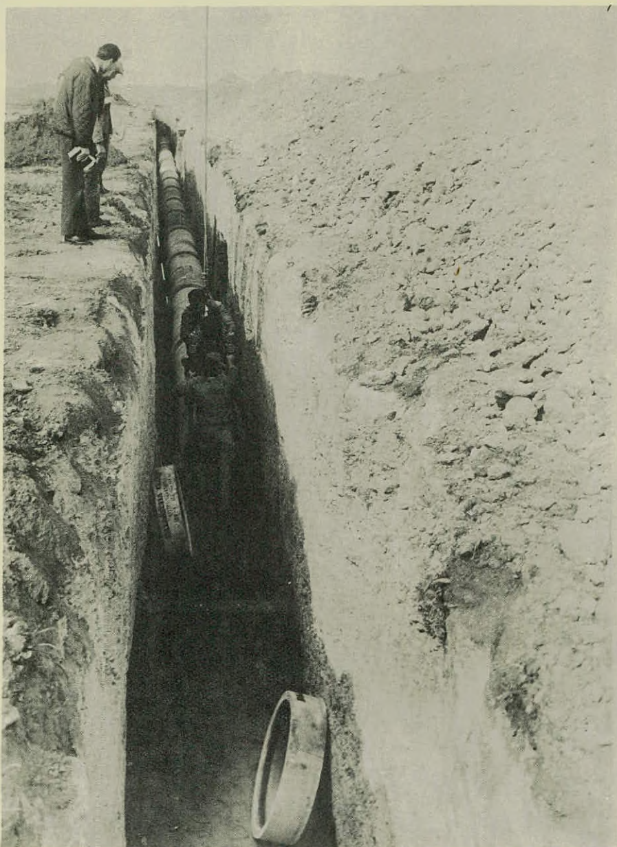
FAMAGUSTA WATER SUPPLY KHIROKITIA-PHRENAROS PIPELINE LAYING OF 650 m.m. dia A.C. PIPELINE
