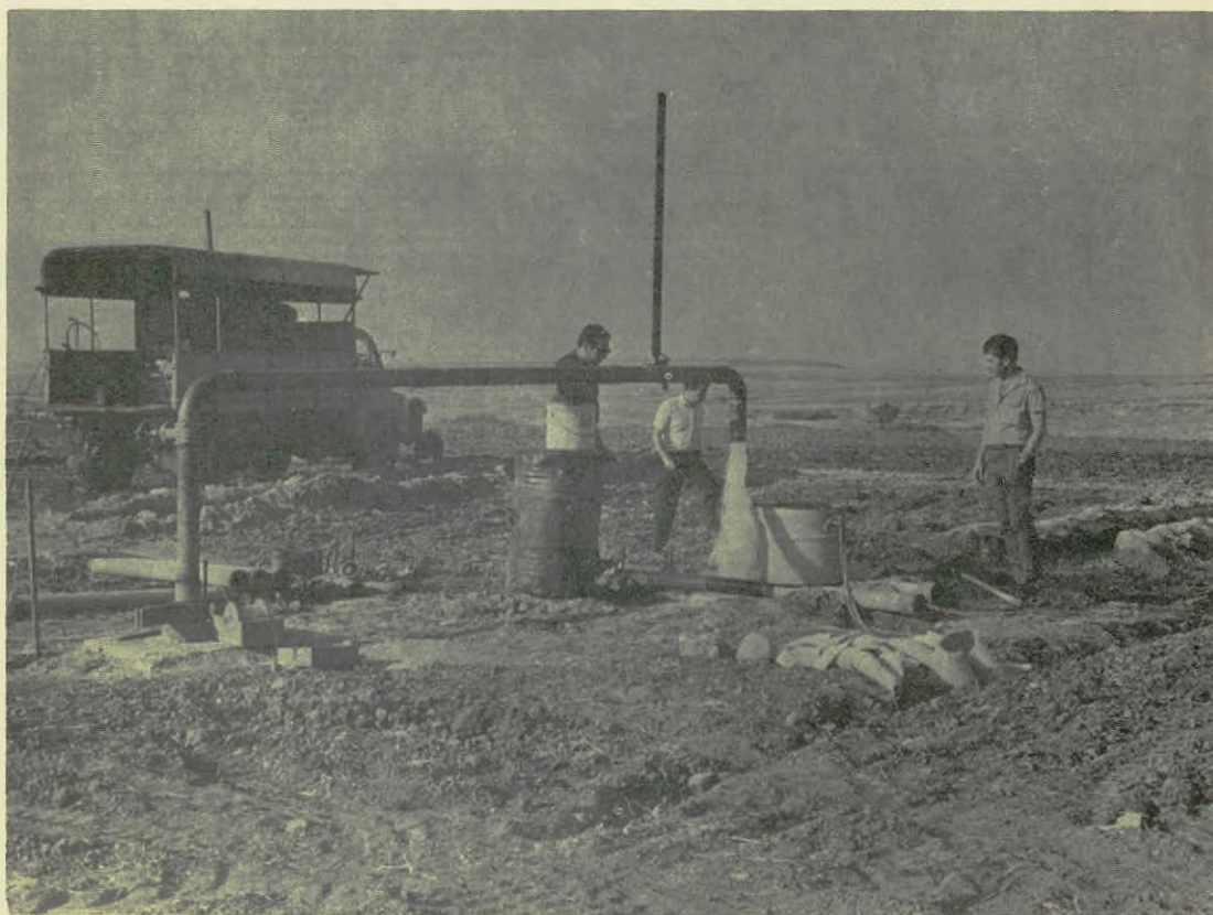
TYPICAL TEST PUMPING OF A NEWLY DRILLED BOREHOLE FOR WATER
