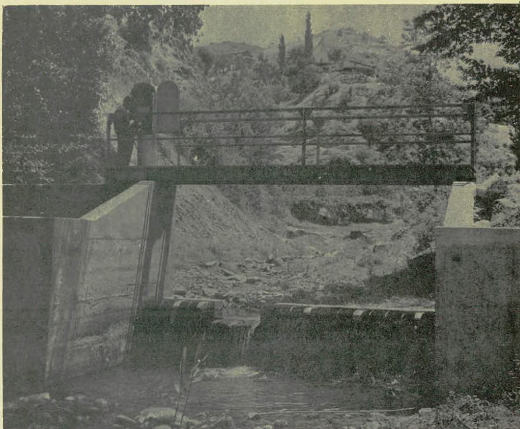
MEASURING WEIR WITH AUTOMATIC RECORDER AT KALOPANAYIOTIS MARATHASA RIVER
