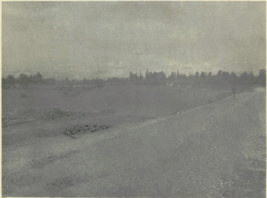
KONDEA RECHARGE DAM Capacity: 18 million gallons. Height :- 20 ft Photo by courtesy of P.I.O. (No 28A 2144)
