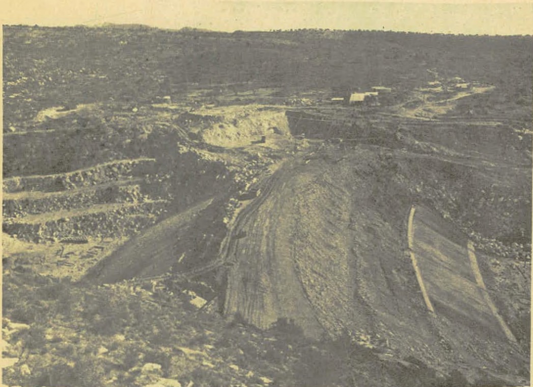
Polemidhia dam. When completed in summer 1965, the Polemidhia dam will be the largest in impounded capacity i.e. 750,000,000 gallons or 3,400,000 metric tons of water. The dam commands 4000 donums in the Limassol area of mainly orchards.
