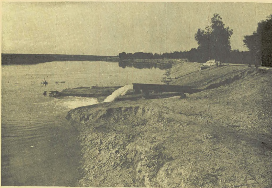
Ayios Loucas lake (Famagusta). 2 No. pumps with an output of 50,000 gallons per minute each are discharging the Sweet water lake waters into the Ayios Loucas lake which are in turn directed by tunnel to the Ayios Memnon spreading grounds.
