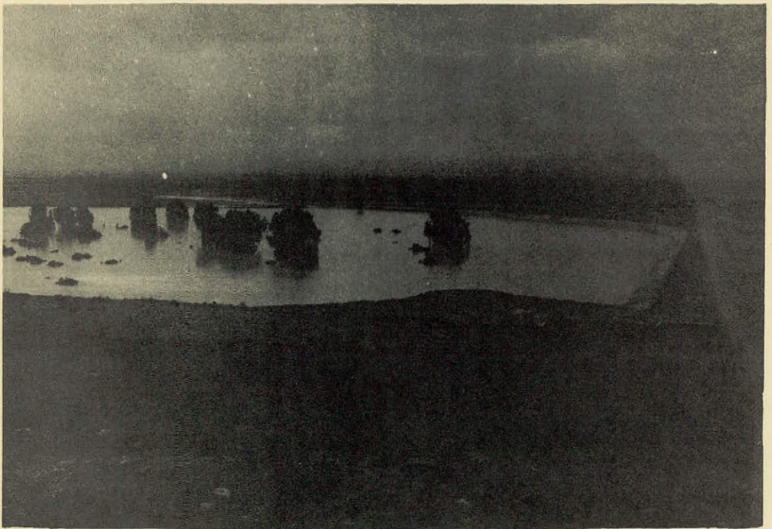
Ovgos dam, is 46 feet high and can impound 195 million gallons of water, thus commanding 3,000 donums of vegetables and orchards.
