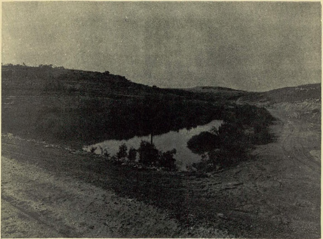
Paralimni Panayia dam (Famagusta). The pictured dam is one of the many constructed in the Famagusta area with the purpose of replenishing the depleted aquifer in the area. Panayia dam has a capacity of 10 million gallons.
